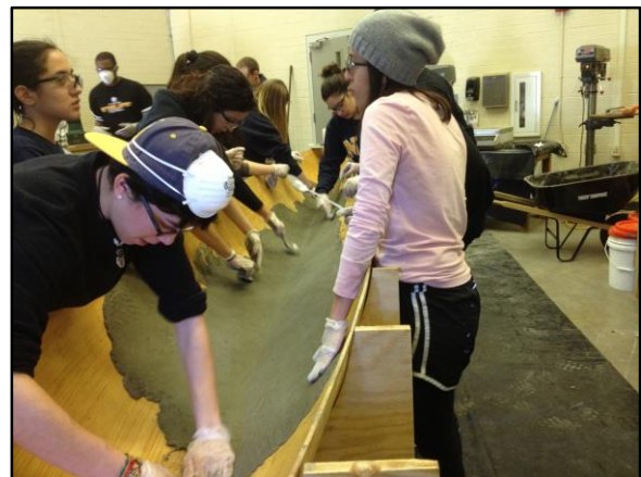
Figure 8: Application of first 1/8 inch layer
